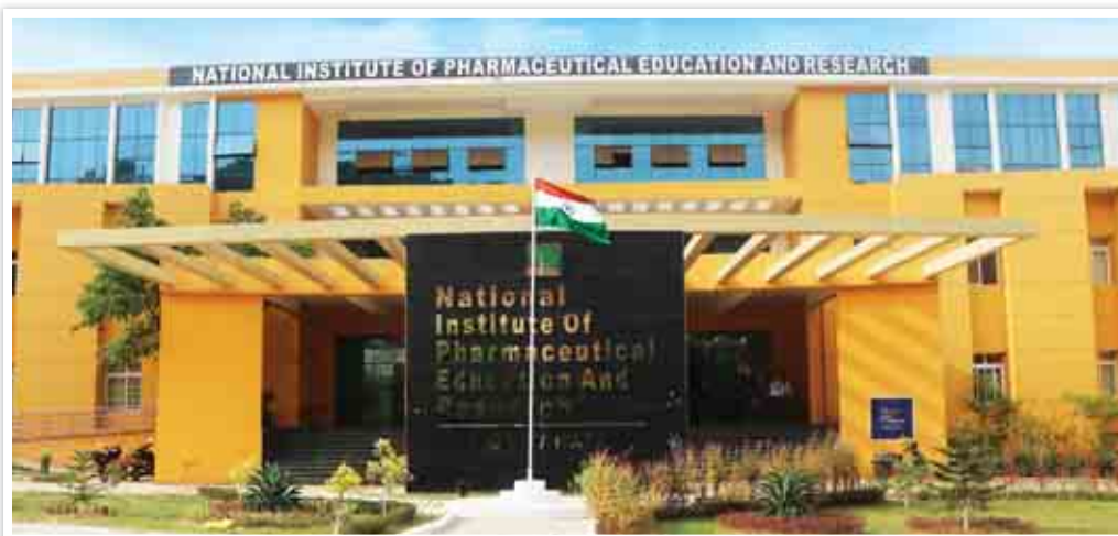
Main Entrance (Admin Block)
